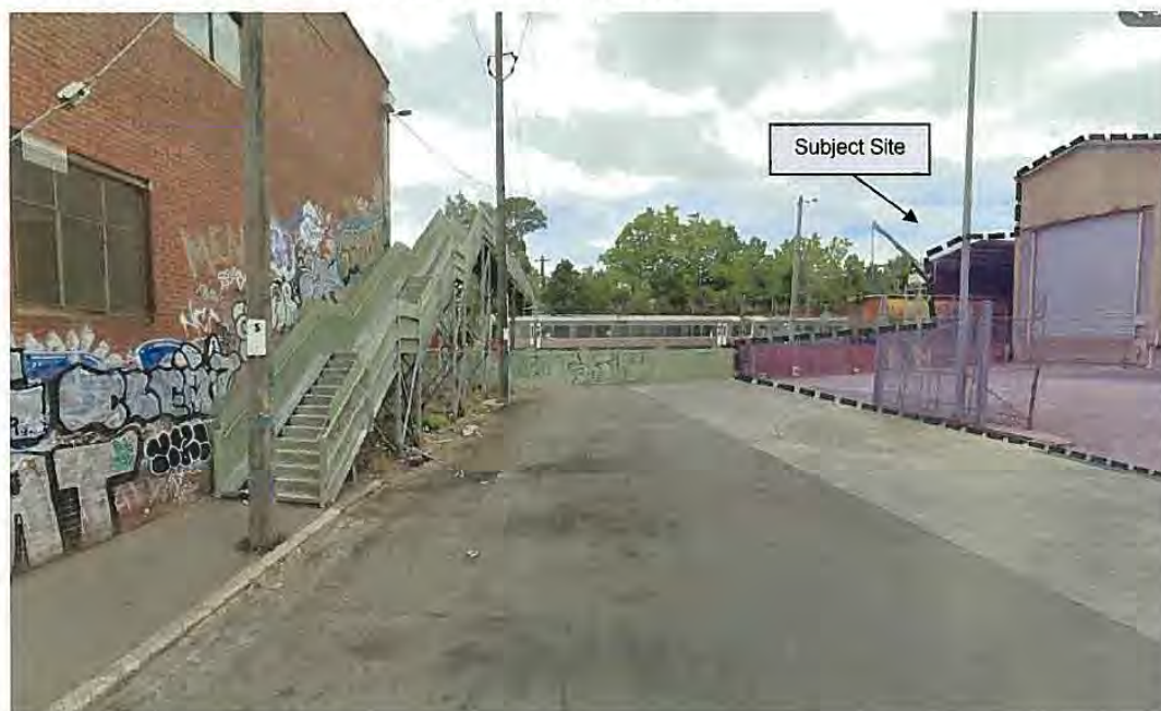
Figure 20: Existing Arden Street Pedestrian Bridge Approach
