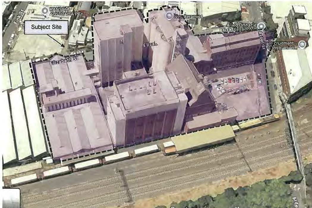
Figure 21: Existing Rail Corridor Site Interface
